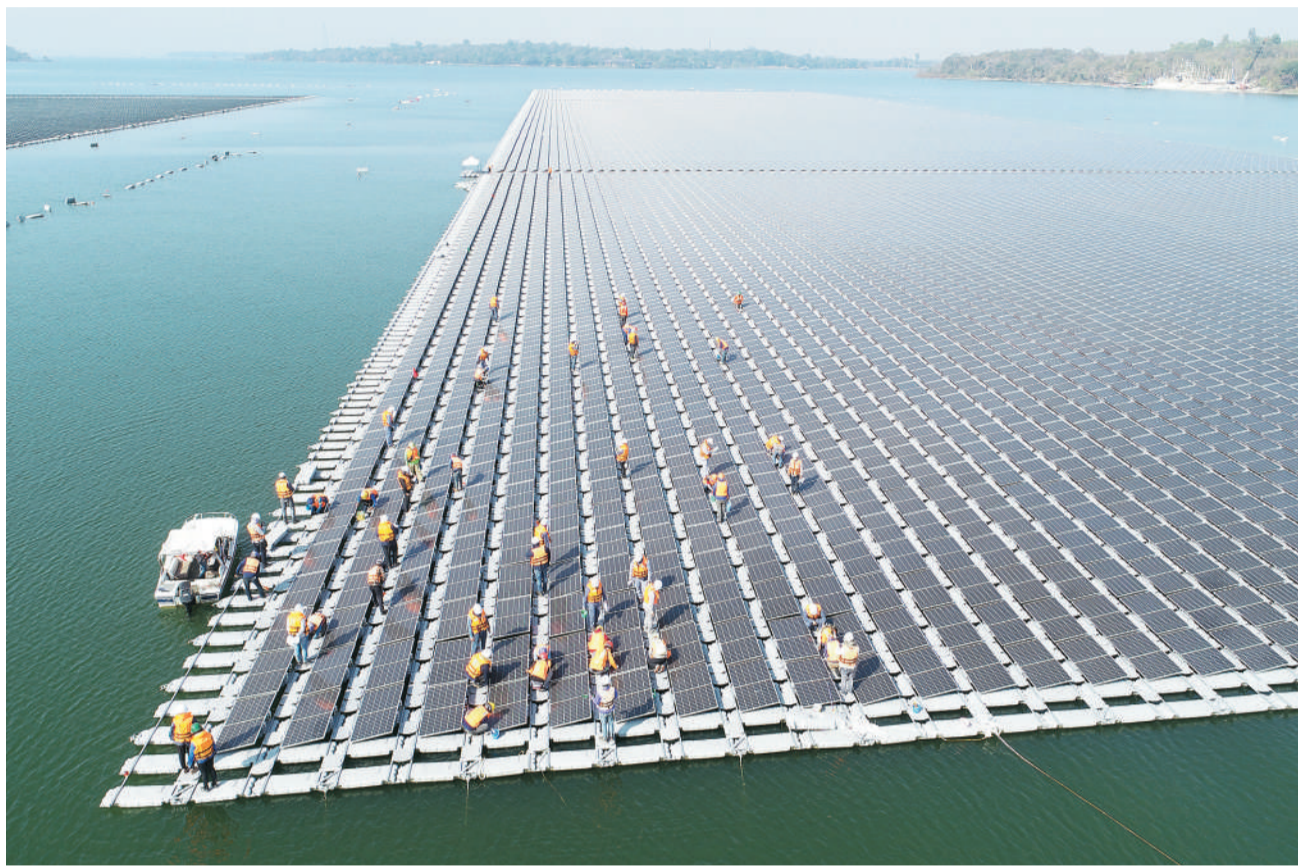
Construction workers checking the installation of floating solar panels at Sirindhorn Dam in Thailand's northeastern province of Ubon Ratchathani. The project is jointly constructed by China and Thailand. (PHOTO: XINHUA)
